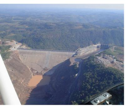
Damage to upstream side of Campos Novos Dam in Brazil after uncontrolled emptying of reservoir. This 880 MW completed project is seeking CDM validation.
