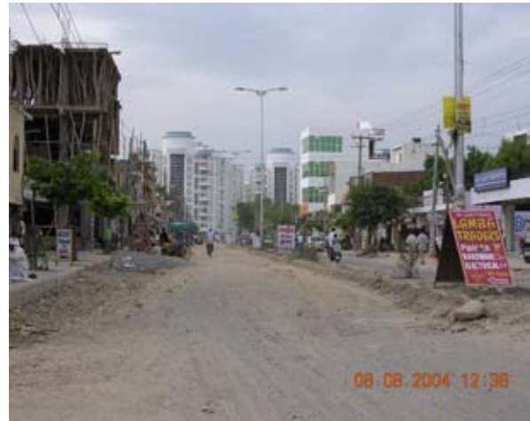
UP-UAH and UP-UAE under construction , re-construction and re-development
