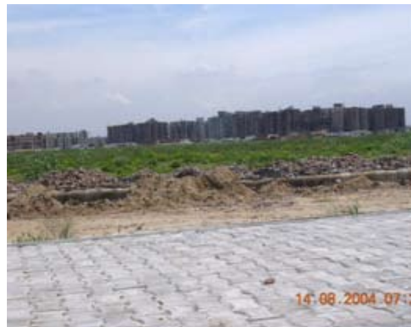
Construction of related infrastructure
