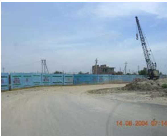
Construction of the Delhi Metro Corridor and related facilities
