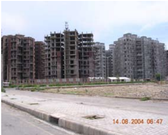
P-CH under construction
