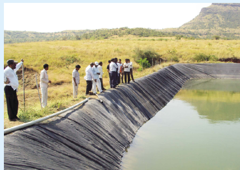
Water tank with polythene sheet in the bottom
