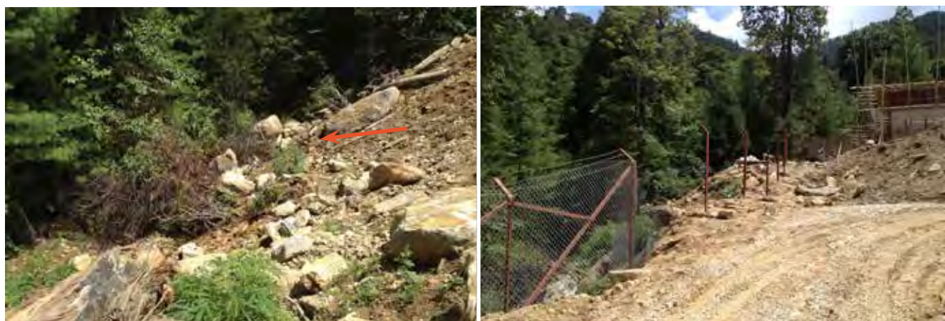
(a) Excavated soils and rocks dumped downslope toward creek perimeter; (b) fence only just being installed 17 months after project start, precluding the work needed to stabilize the western perimeter of the site.
