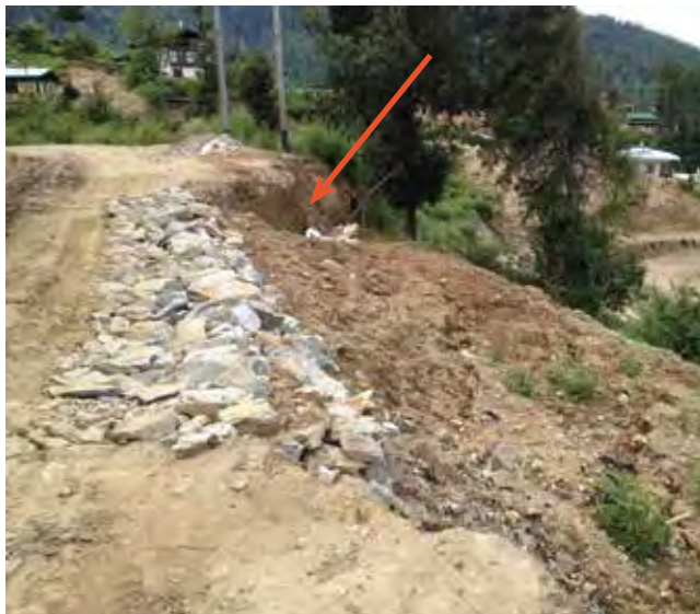
Figure 12: Failure of the Road near the Water Treatment Plant Site in Chamgang
