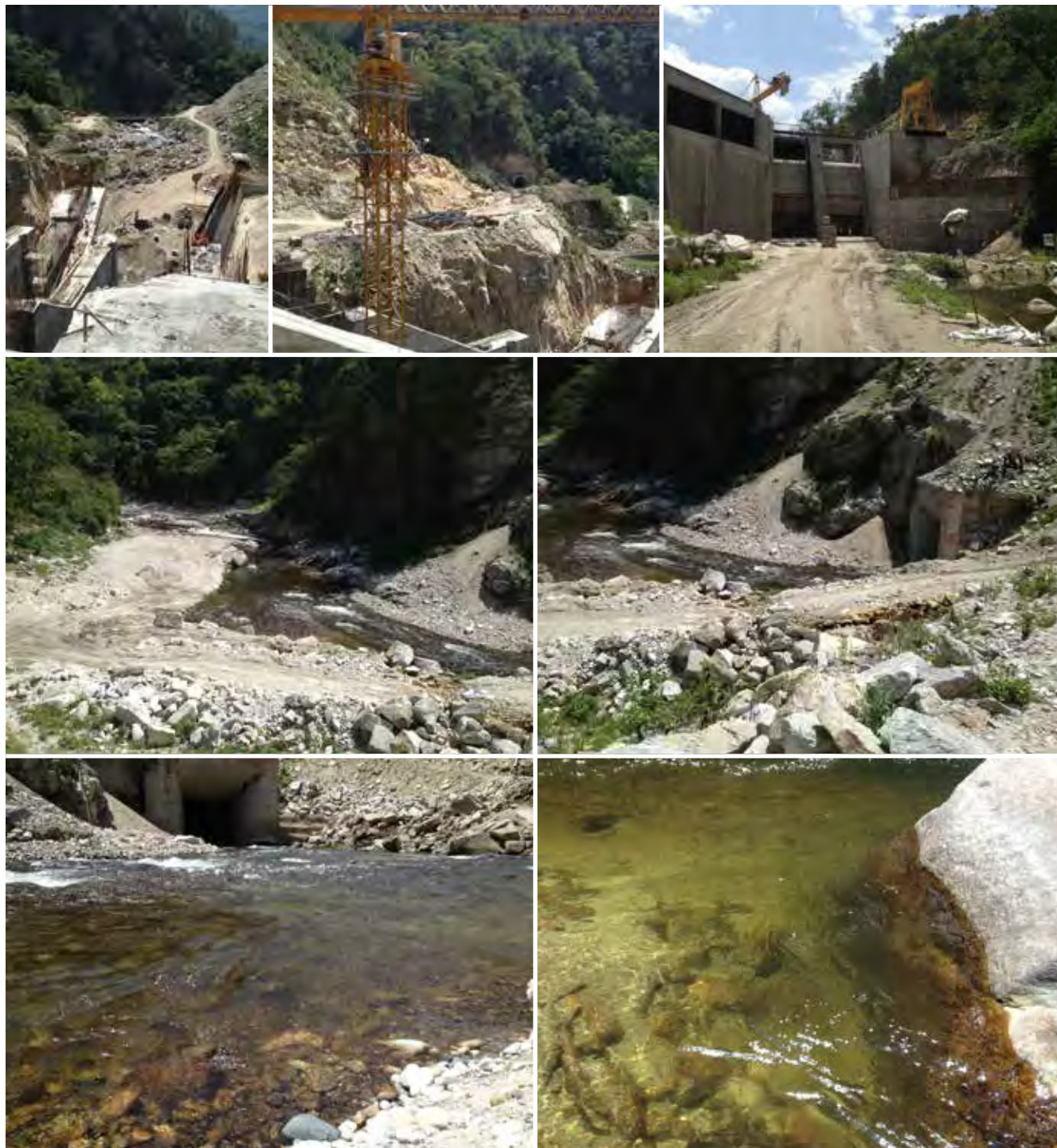
L-R, top-bottom: (a) Downstream of dam; (b) beginning of headrace tunnel; (c) gates and intake; (d) upstream of cofferdam; (e) diversion flow tunnel; (f) inflow to flow diversion; (g) excellent water quality near diversion tunnel.
