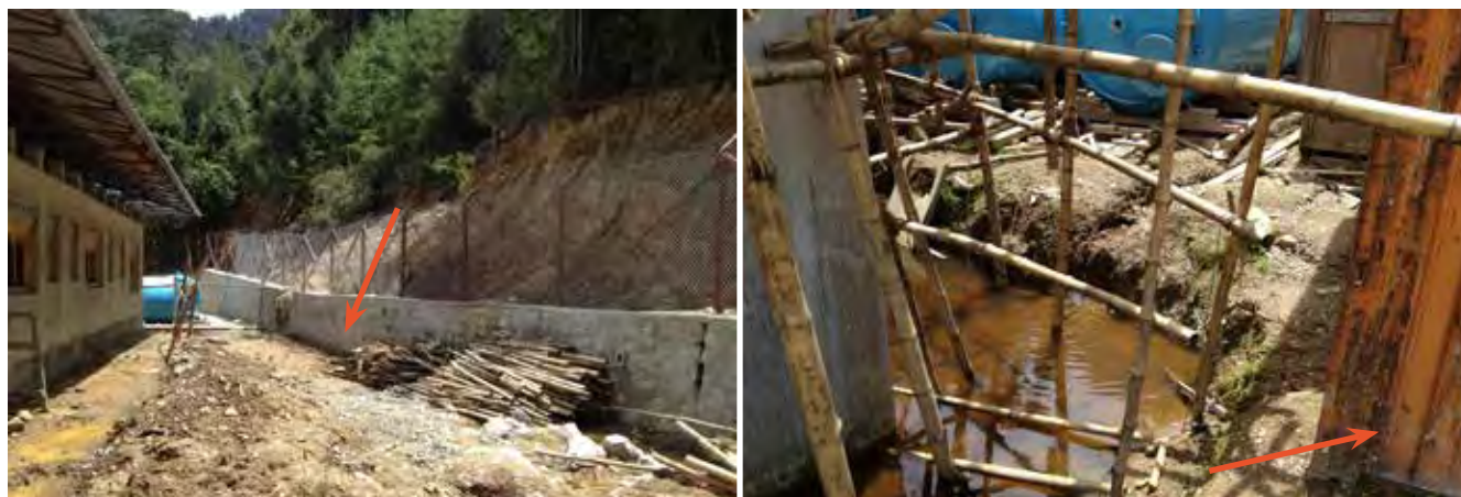
Figure 7: Site Drainage Issues around Structure Footings in Chamgang
