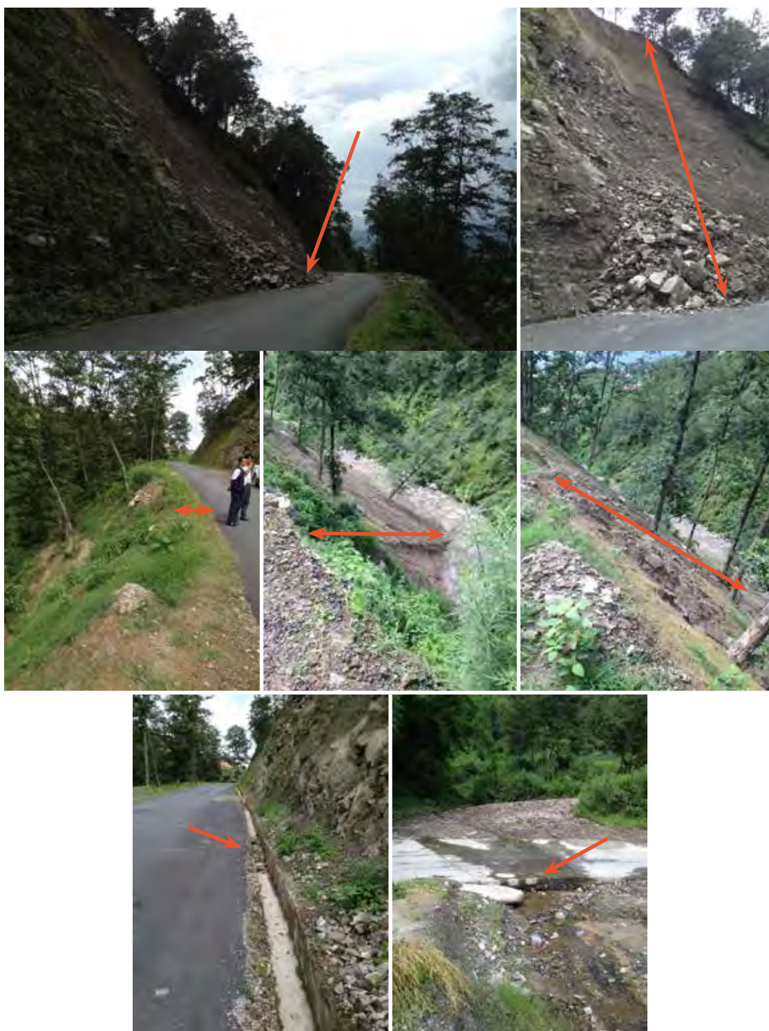
Figure 40: Steep Slope and Rockfall on the Nala Road
