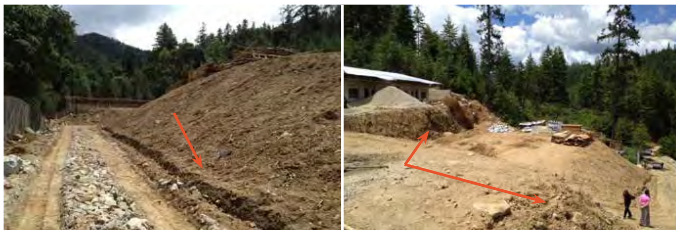
Figure 5: Exposed Slopes at the Water Treatment Plant Site, with Temporary Drainage Ditches in Chamgang
