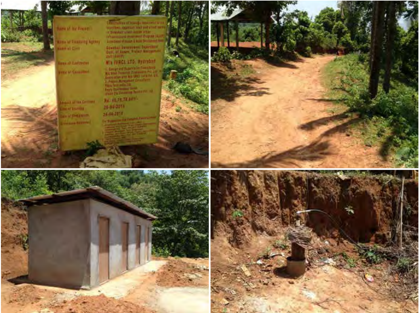
L–R clockwise: (a) Signage for site details (facing the wrong way); (b) access road (some tree clearing will be required, as well as widening and regrading); (c) newly drilled tubewell for water supply for the construction site; (d) newly constructed toilets for the laborer camp.
