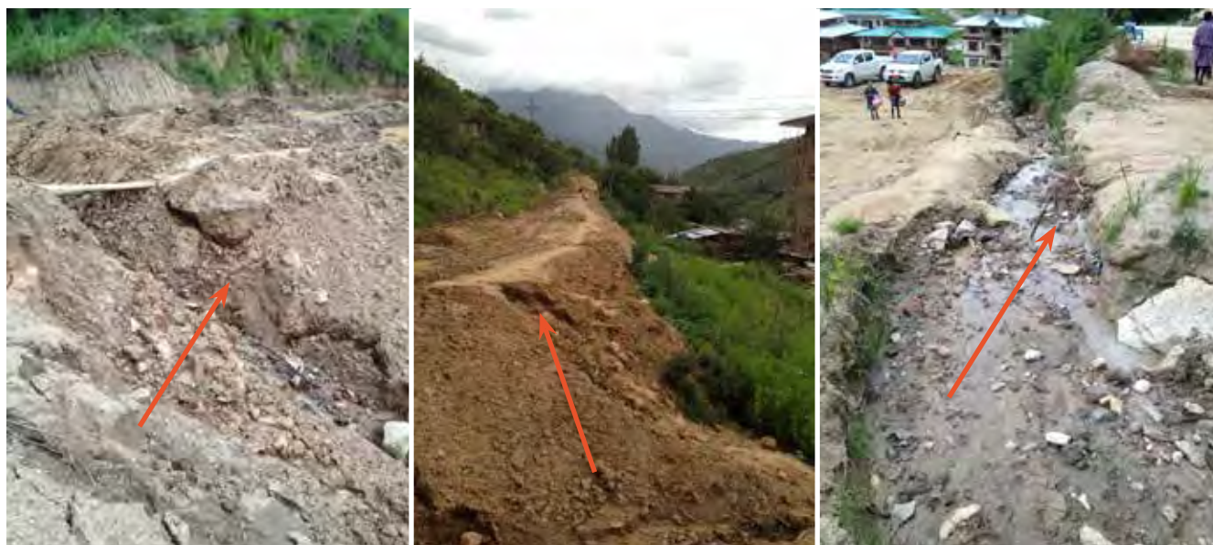
Figure 15: Gully Erosion and Incipient Slope Failure in Some Locations in Changbangdu
