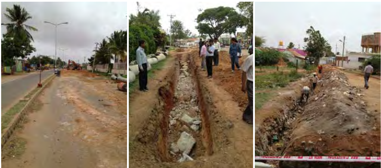
Figure 29: Sewage Pipe Trenching in Town
