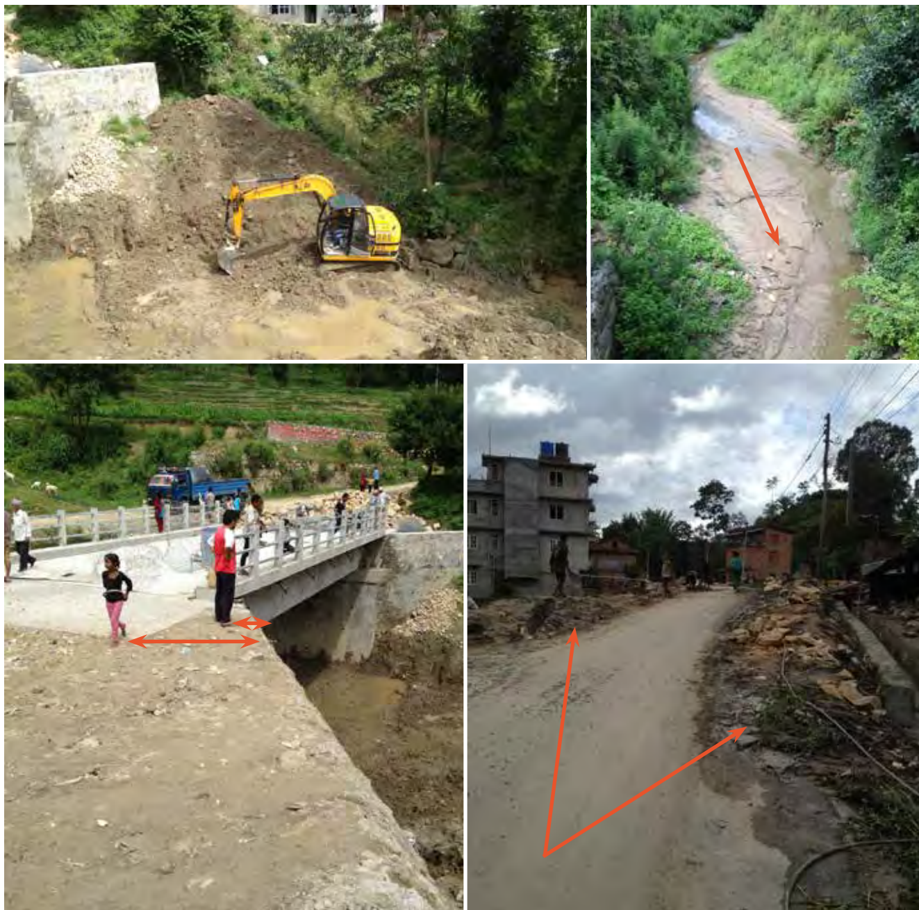
Figure 41: Realignment of the River under the New Bridge on the Nala Road
