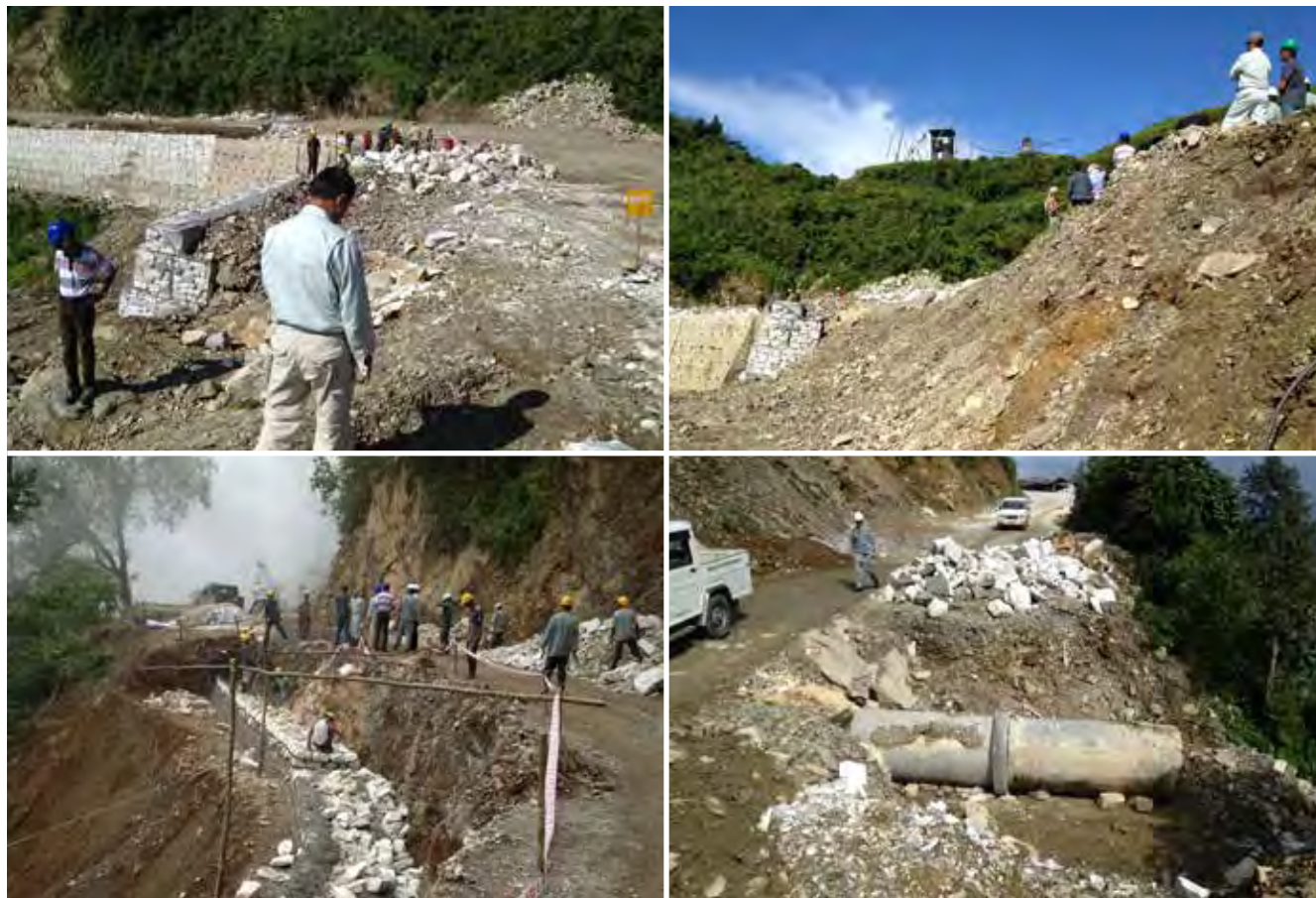
Figure 18: Cross-Road Drainage and Retaining Walls Task-Sequenced to Reduce Road and Slope Failure Risks in Manitar–Raidak Section
