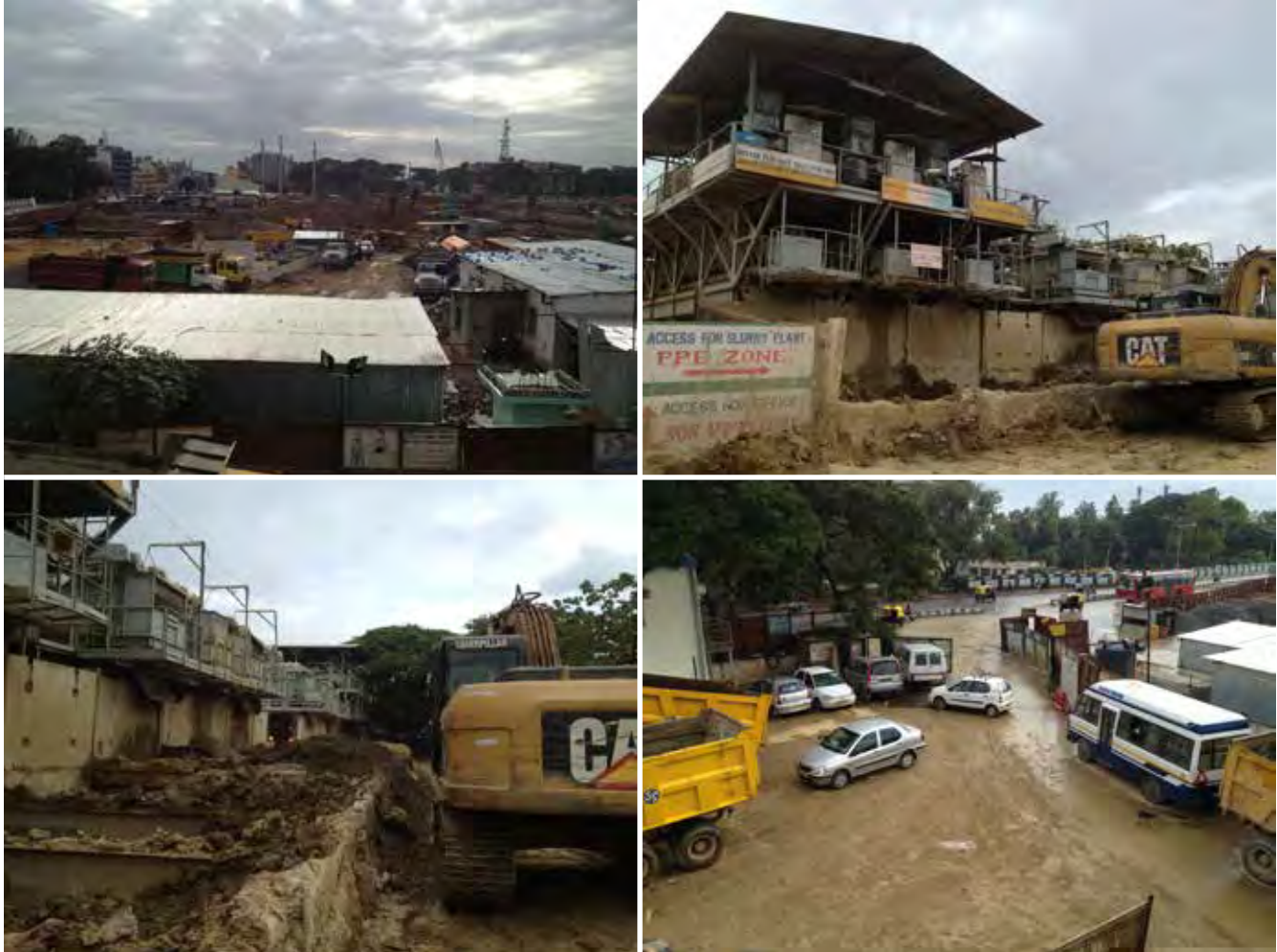
L–R: (a) Intersection of north–south and east–west lines; (b) massive surface excavation and tunneling; (c) slurry plant, sediment separation, and trucking off-site (to MS Palya); (d) no sediment controls at site perimeter.
