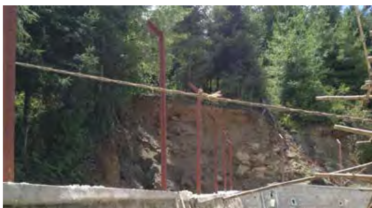
Figure 9: Unstable Cut Slope behind Retaining Wall in Chamgang
