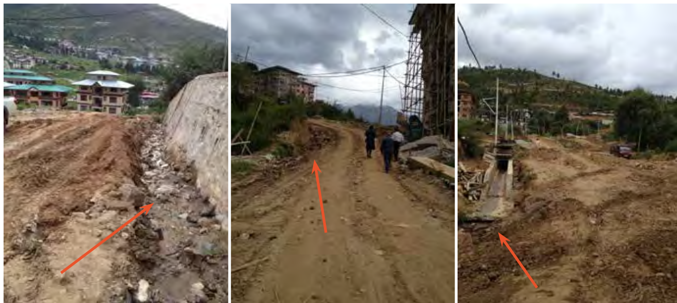
Figure 14: The Main Issues Are Significant Amounts of Loose Exposed Sediments and Challenging Site Drainage on a Very Steep Slope in Changbangdu
