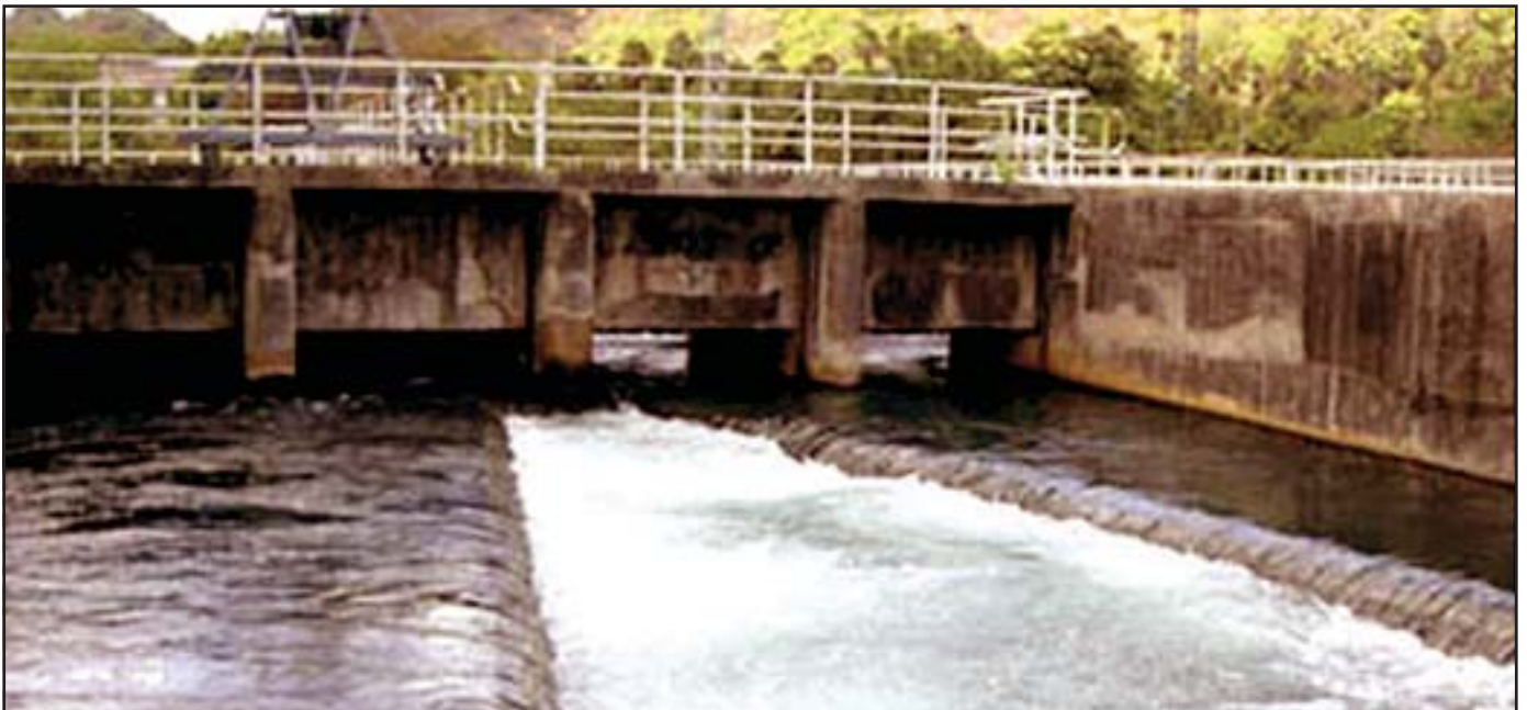
Figure 5: WORLD-CLASS WATER... BMC's water treatment plant at Bhandup; the largest facility in Asia.
