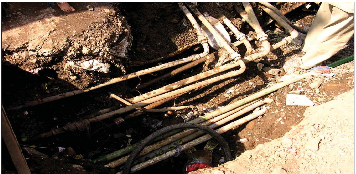
Figure 10: SPAGHETTI PIPELINES IN SLUMS... Will expensive water meters work here? [Source: BMC 2010]
