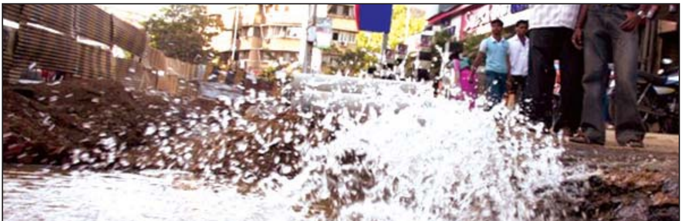
Figure 6: DOWN THE DRAIN... Mumbai loses millions of liters of water through pipe bursts, a common occurrence on Mumbai’s old and weak distribution network. [Source: www.timesofindia.indiatimes.com ]
