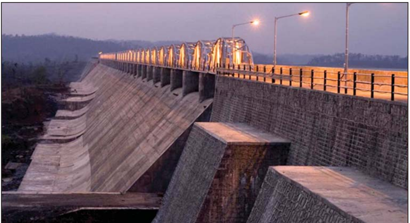
Figure 4: ENGINEERING MARVEL... Tansa Dam, built by the British in 1925. The dam’s height was raised and its structure strengthened for any tectonic eventuality indigenously by BMC engineers. [Source: www.magicalmumbai.com ]
