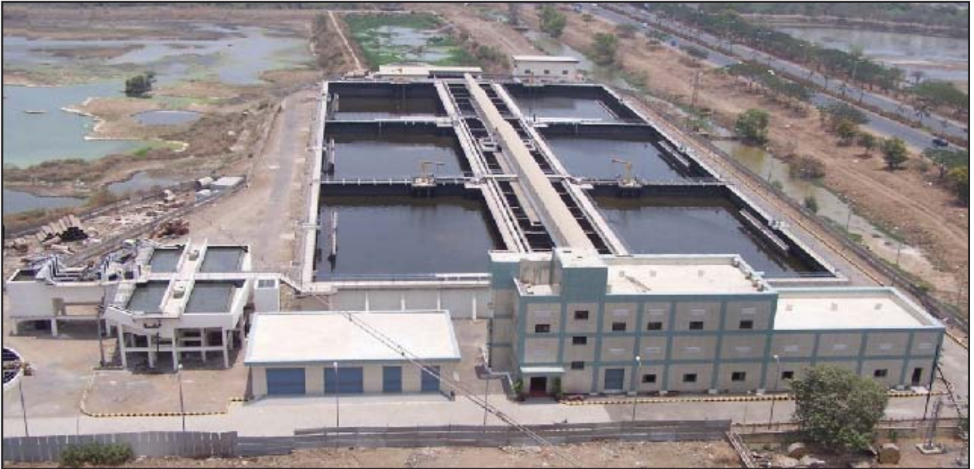
Figure 17: FROM BLACK TO BLUE... The NMMC's Sewage Treatment Plant at Nerul. The plant has an ultimate capacity of 100 MLD. [Source: NMMC]
