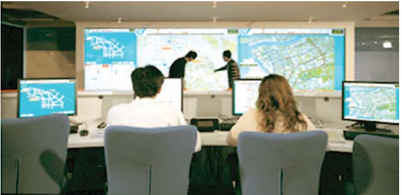
Figure 23: REMOTE CONTROL... GIS maps of the utility pipes in PVWC's control room give real-time information and data. [Source: Paper on Best Practises in Water Supply in Pudong, Shanghai, presented at Zaragoza Water Expo, 2008]
