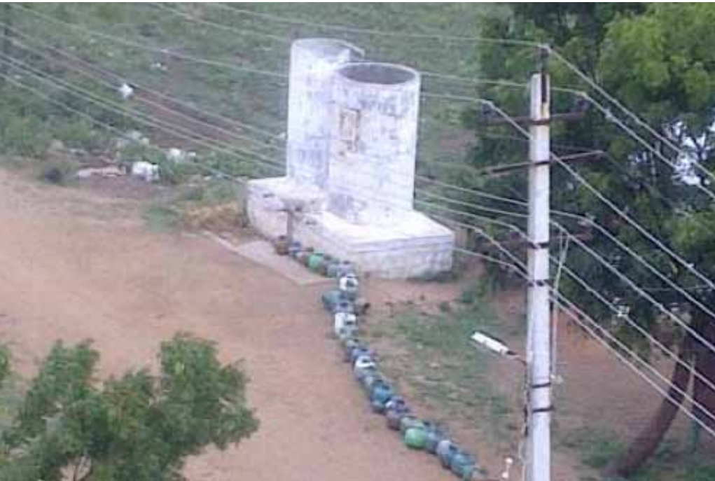
Before commencement of 24/7 water supply, many people in Ilkal used to receive water only once every 2-5 days. Hence, people who queued up for water kept their pots at the cistern.
