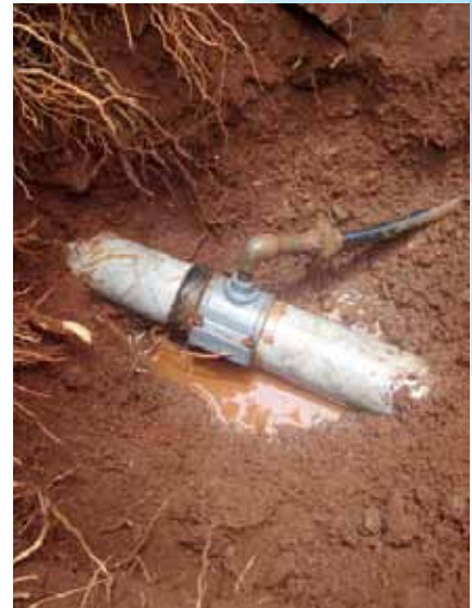
New house service connection over polyethylene pipe (less prone to leakage).
