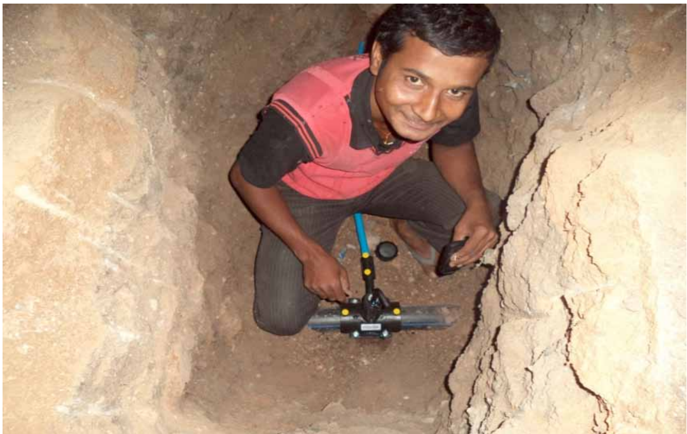
Installation of new house service connection over polyethylene pipe.
