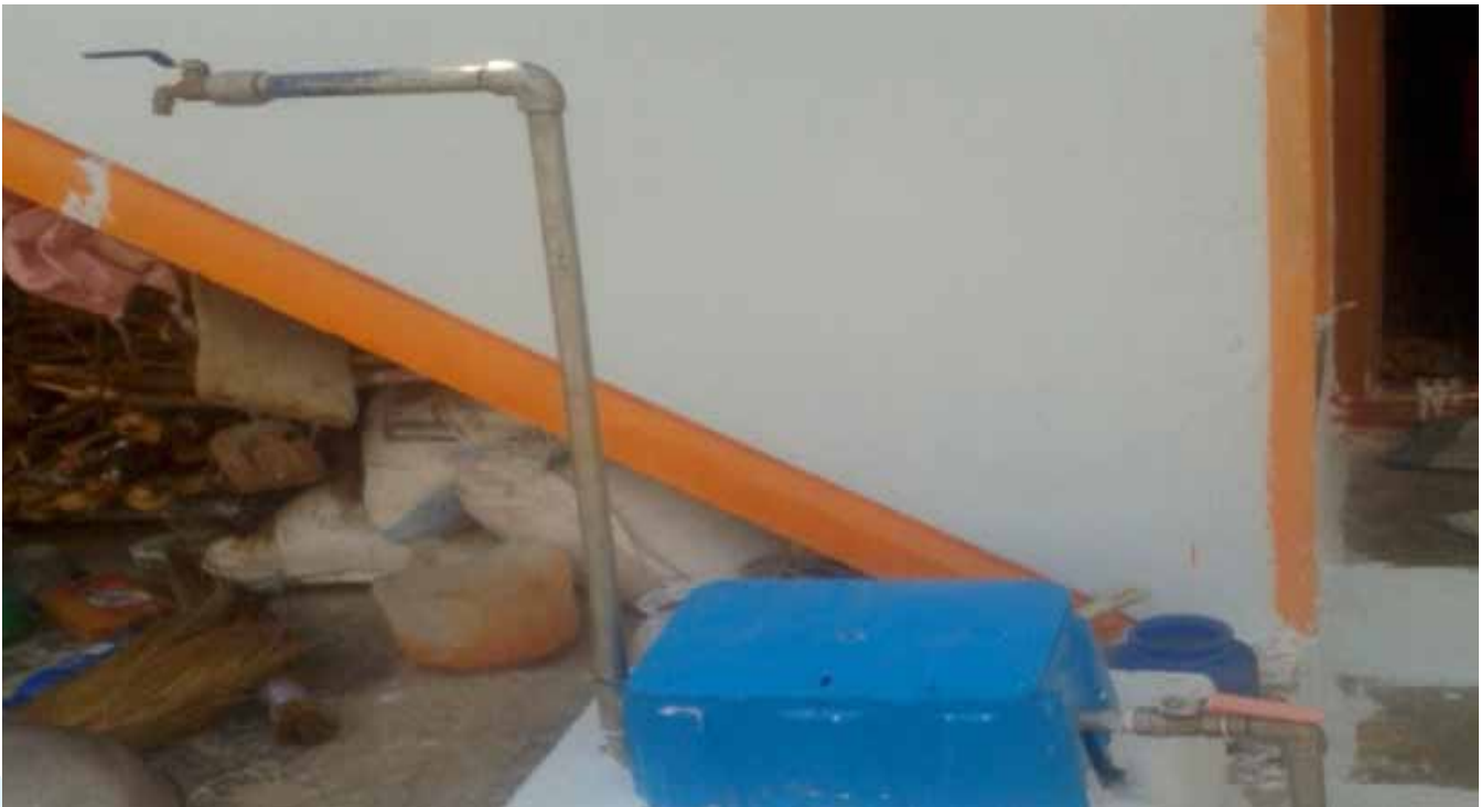
New house service connection.
