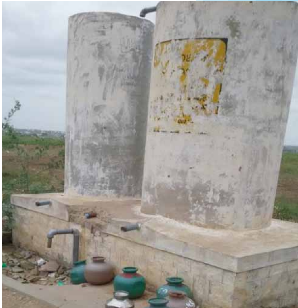
After commencement of 24/7 water supply, queuing up pots at the cistern is no longer necessary.
