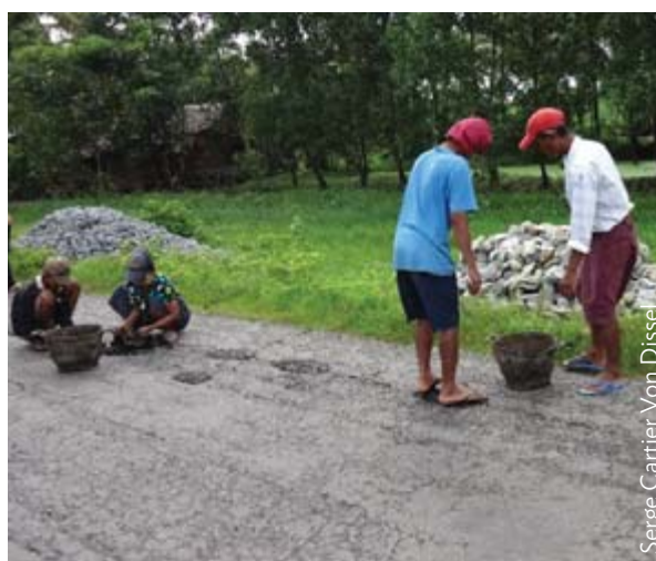
Figure 25: Pothole Patching in Build–Operate–Transfer Contracts
