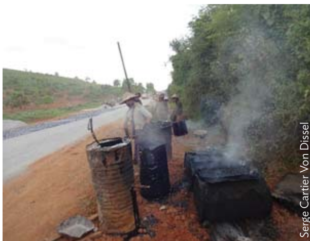
Figure 24: Heating of Bitumen
