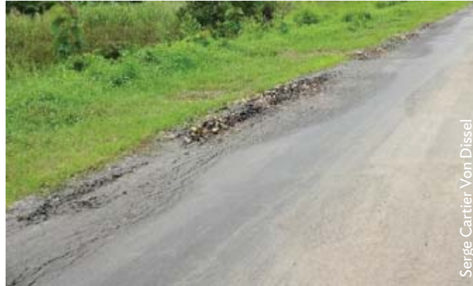
Figure 22: Defects Observed in Widening Works
