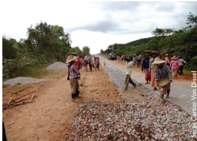
Figure 23: Spreading of Aggregate
