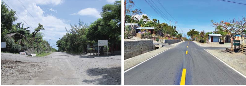
A stretch of road before (left) and after (right) upgrading by the Road Network Development Sector Project
