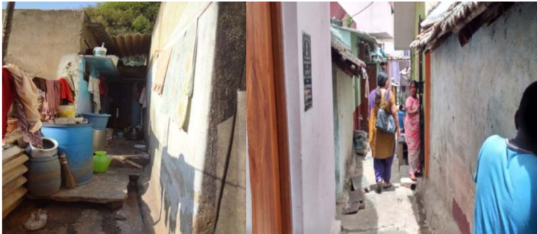
Plate 5: Narrow Lanes and Lack of Space Hinder Construction of Toilets in Swatantrapalya Slum
