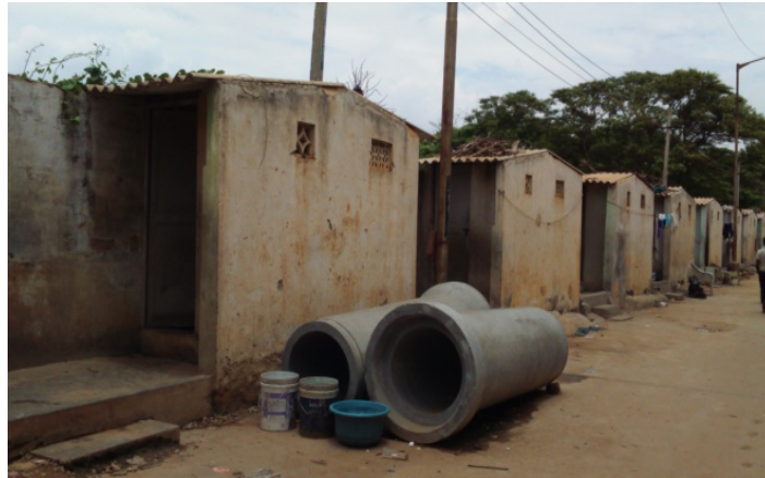
Plate 2: Shared Toilets at Jayaram Slum
