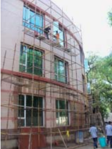
Working at height at RK Khanna Stadium in the last week of July, without safety belts or helmets.
