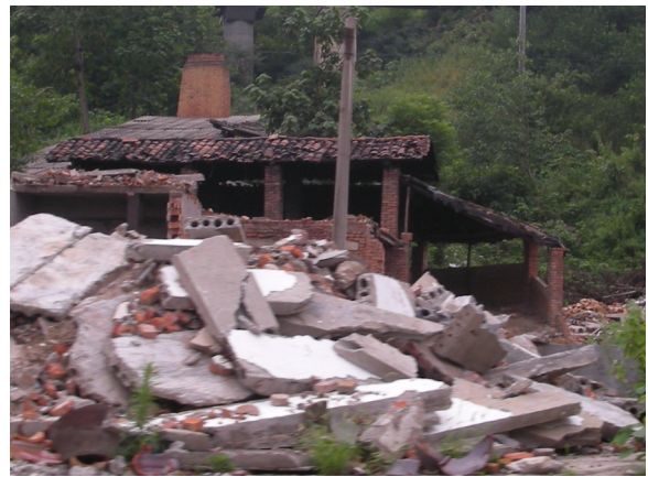
People resettled in the Trial Phase demolished their old houses
